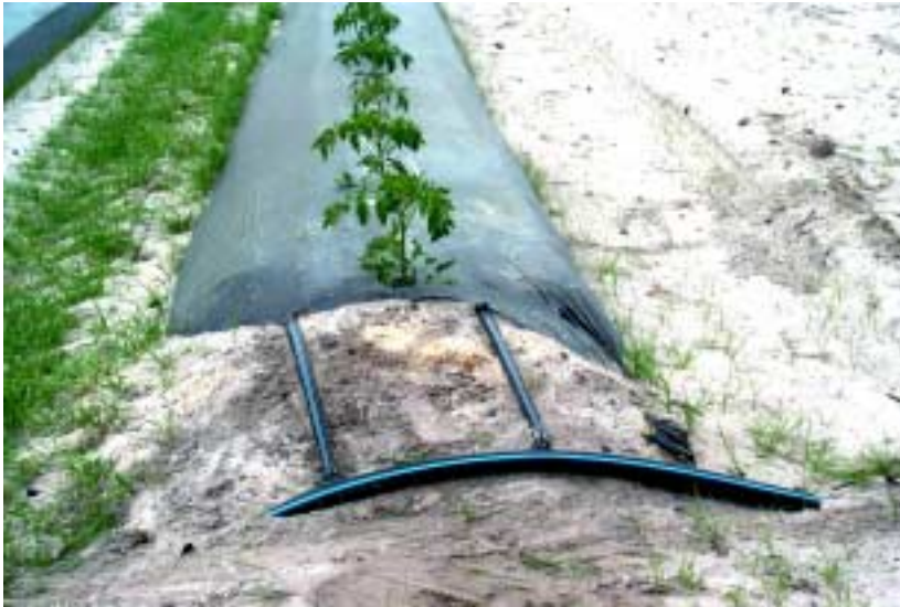
Figure 13: Aqua-TraXX Connection to Oval Hose
